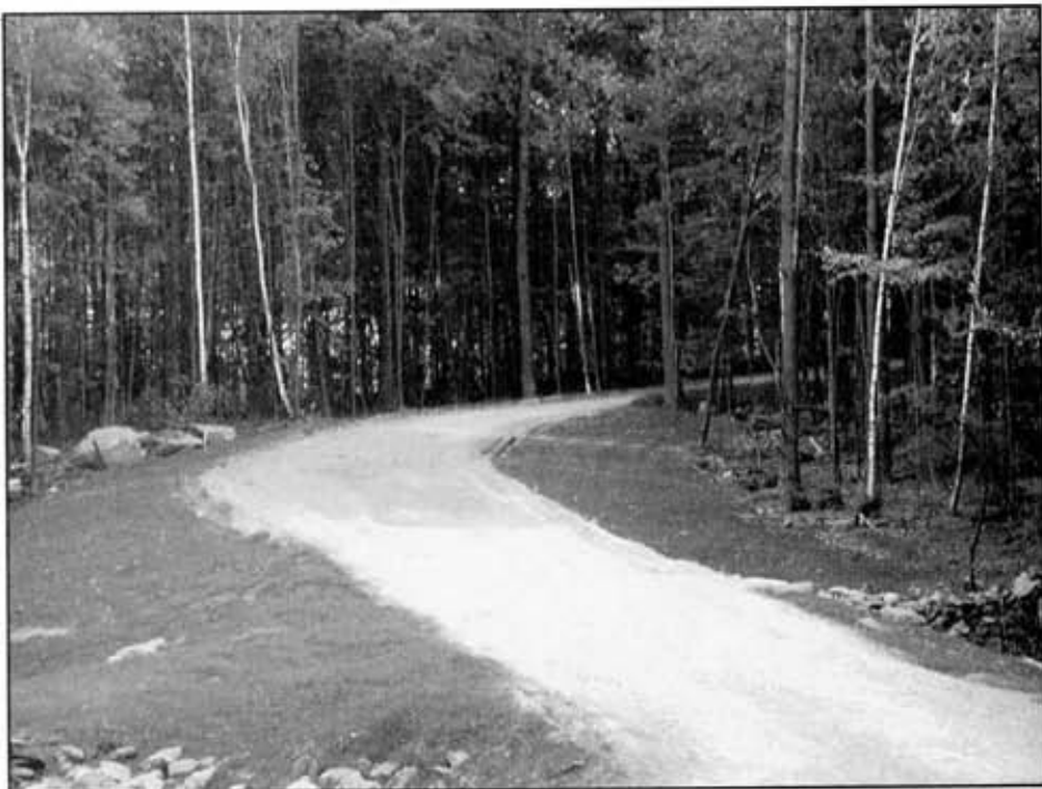
The access road to The Forest Refuge site. This driveway (off Lockwood Rd) was completed in September last year, and follows the same route as the new water line connecting the site to Barre town water. Emergency vehicle access determined the road width, and maximum effort was made to preserve nearby trees.
