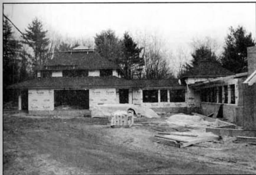
Meditation hall, with roof and framing intact, late Winter, 2002
